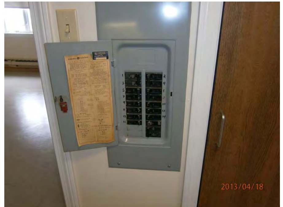
24. Unit circuit breaker panel
