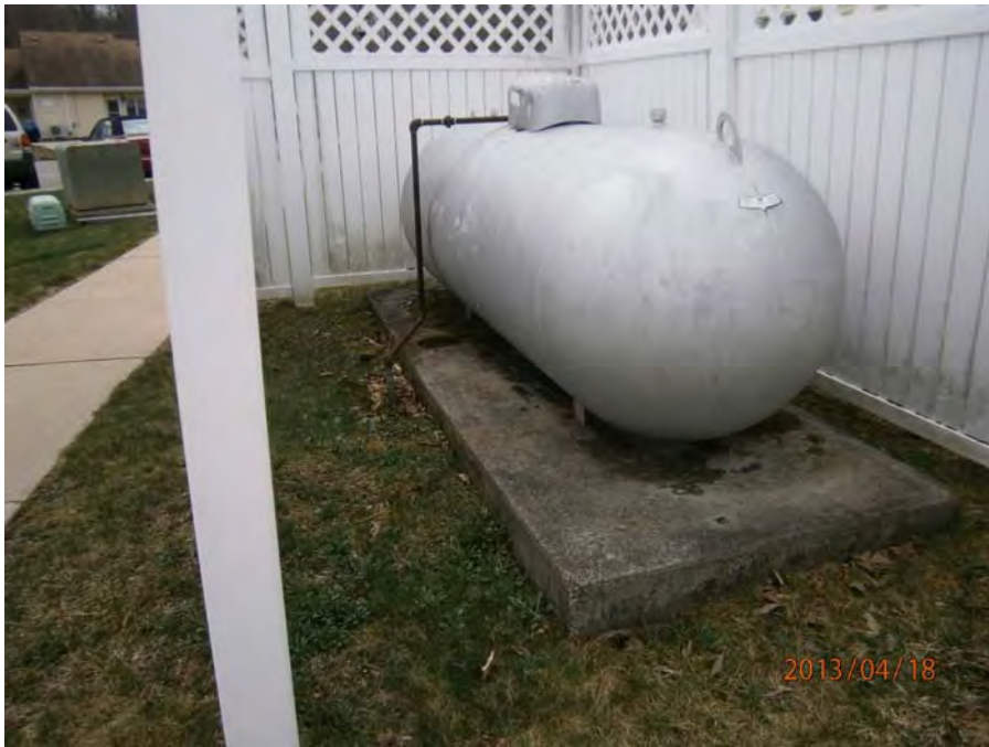
5. Emergency generator fuel tank
