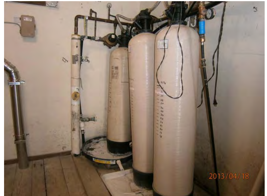
14. Well water treatment tanks
